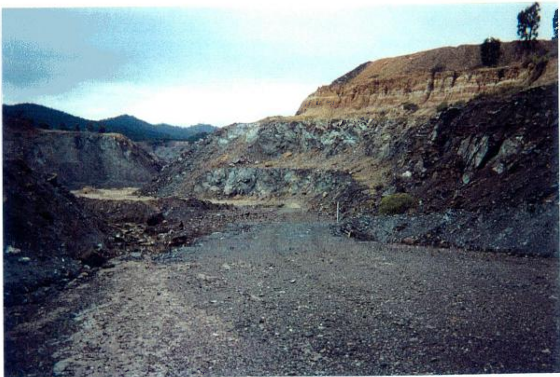
PLATE 2. ROADWAY DOWN TO SOUTH PIT
